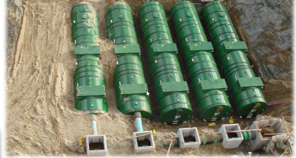
OIL/WATER SEPARATOR BANK INSTALLED AT AN INDUSTRIAL FACILITY FOR STORMWATER DISCHARGE COMPLIANCE AND SPILL CONTROL
