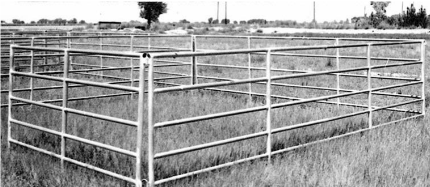
IRON PIPE CORRAL AND HOLDING PEN
