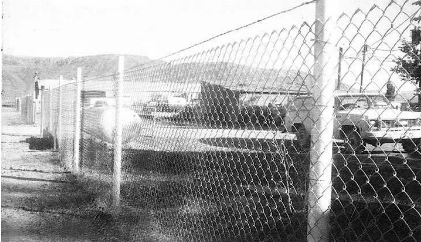
5' CHAIN LINK FENCE NO TOP RAIL
