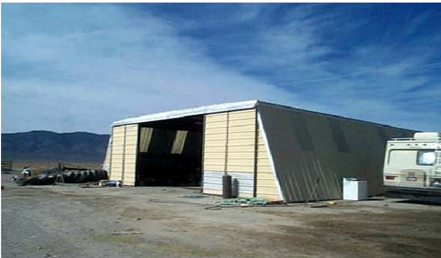
METAL SHOP– SLANT WALL
