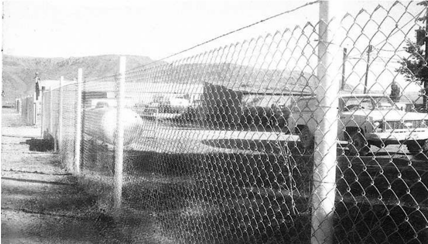
5' CHAIN LINK FENCE NO TOP RAIL
