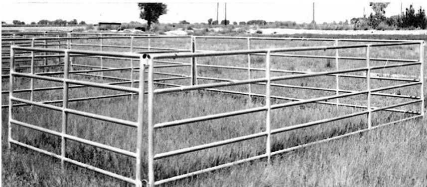
IRON PIPE CORRAL AND HOLDING PEN
