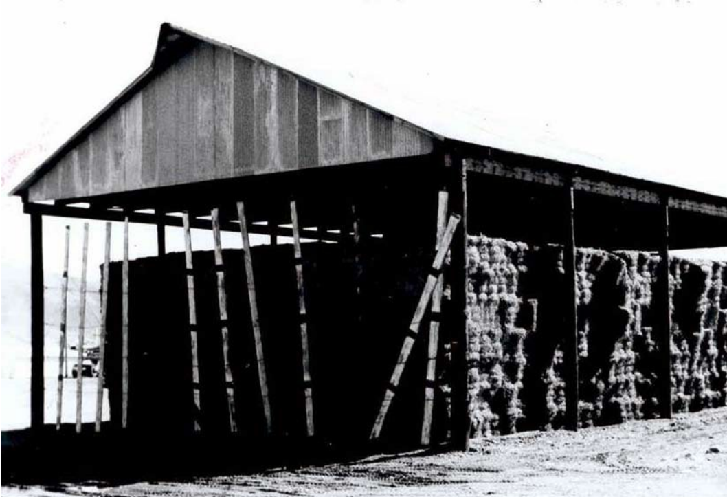
AVERAGE QUALITY – ALL SIDES OPEN WOODEN POLES – WOOD FRAME
