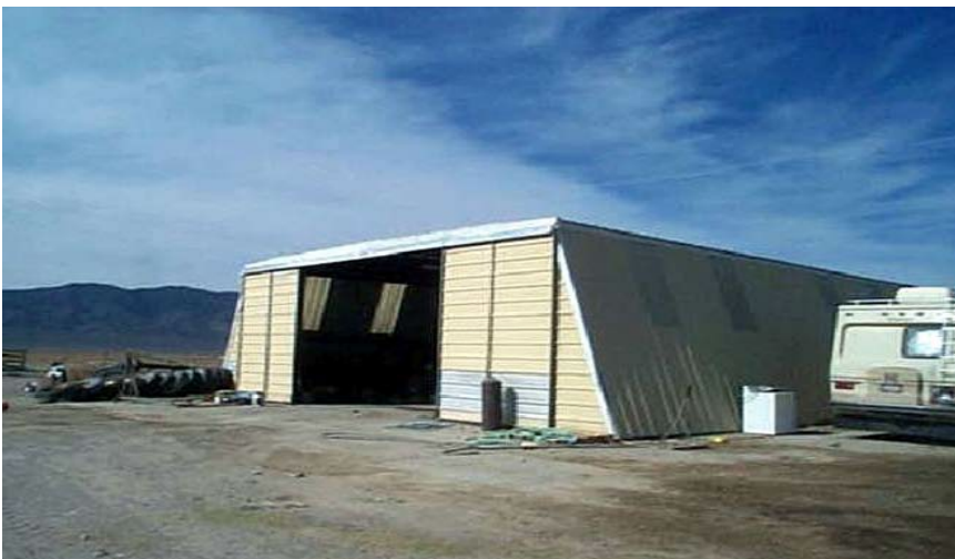
METAL SHOP– SLANT WALL
