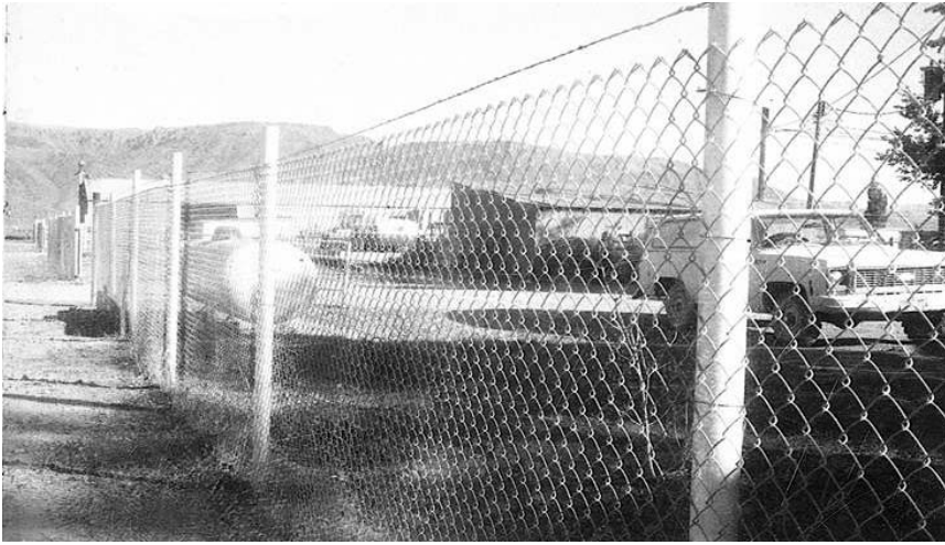
5' CHAIN LINK FENCE NO TOP RAIL
