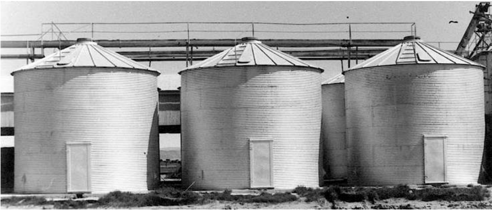
GRAIN STORAGE BINS with CONVEYOR
