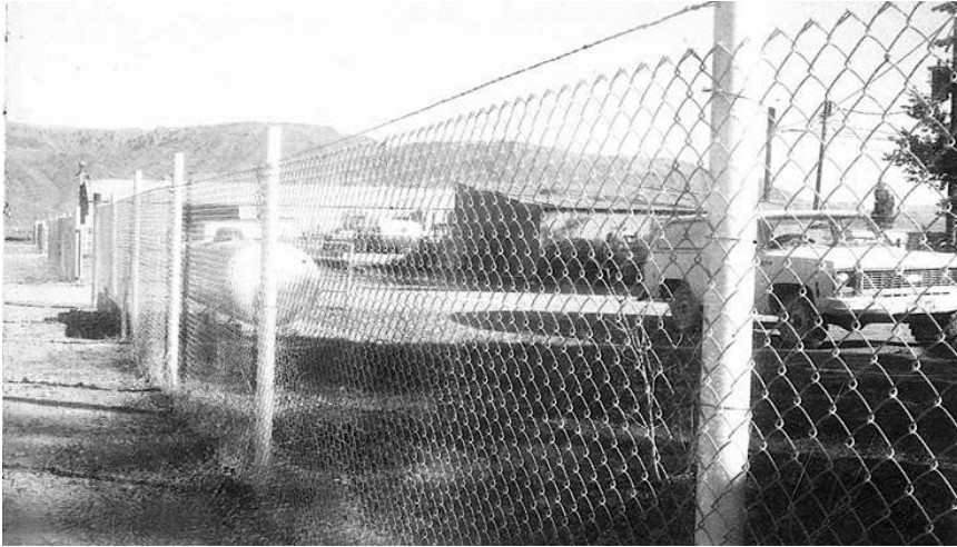
5' CHAIN LINK FENCE NO TOP RAIL
