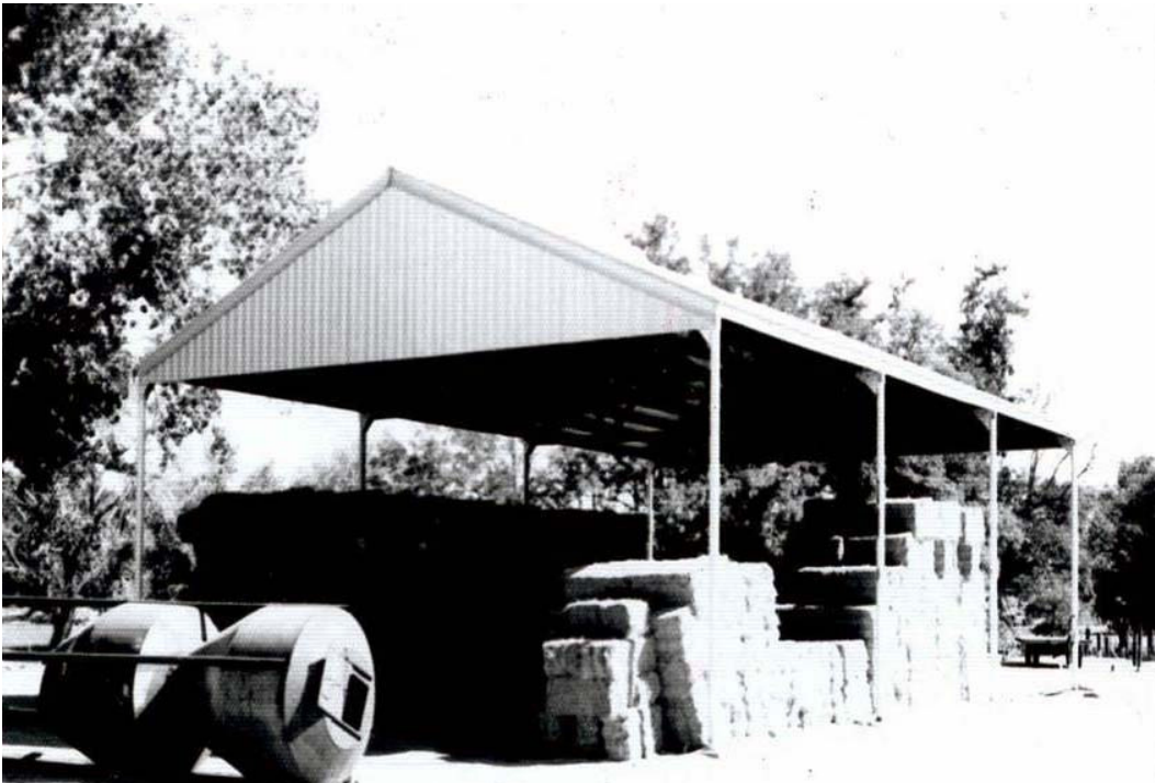
GOOD QUALITY – ALL SIDES OPEN STEEL POLES, STEEL TRUSS & STEEL FRAME
