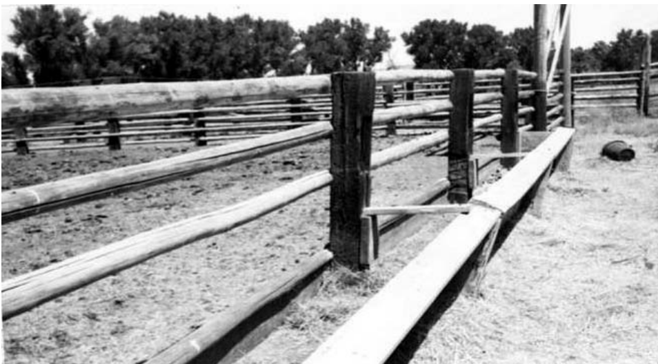
RAILROAD TIE POSTS POLE RAIL FENCE WITH FEED TROUGH AVERAGE QUALITY
