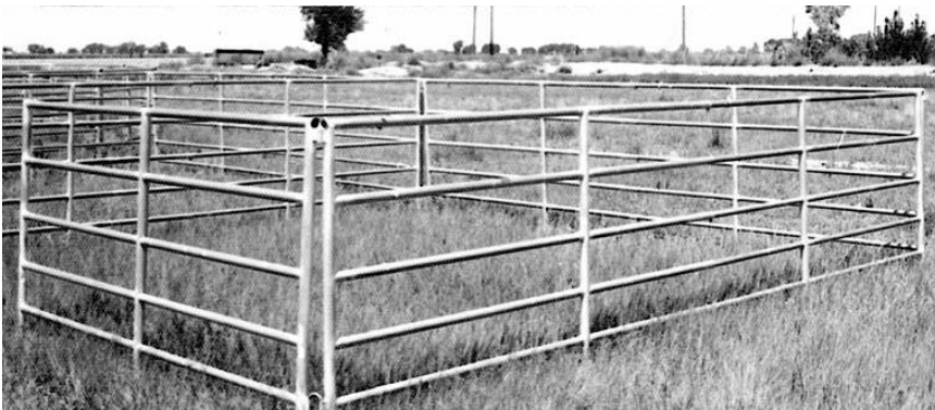
IRON PIPE CORRAL AND HOLDING PEN
