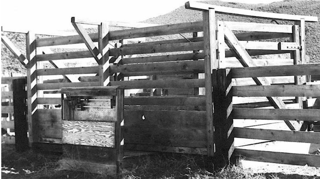
LIVESTOCK SCALE with WOOD CAGE
