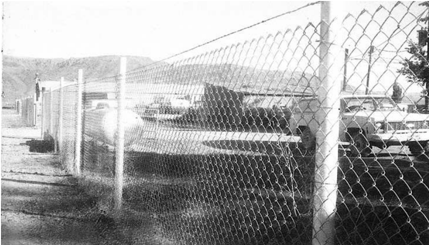
5' CHAIN LINK FENCE NO TOP RAIL
