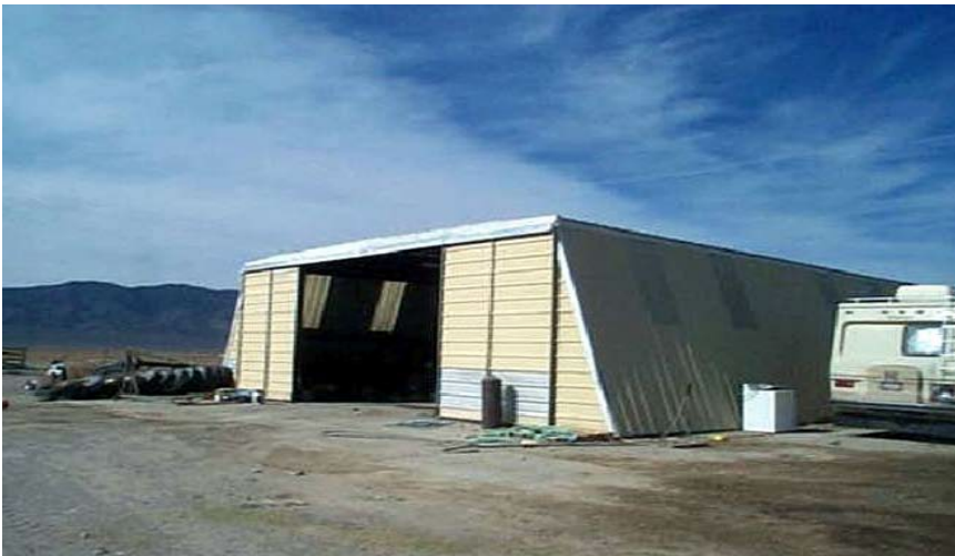
METAL SHOP– SLANT WALL
