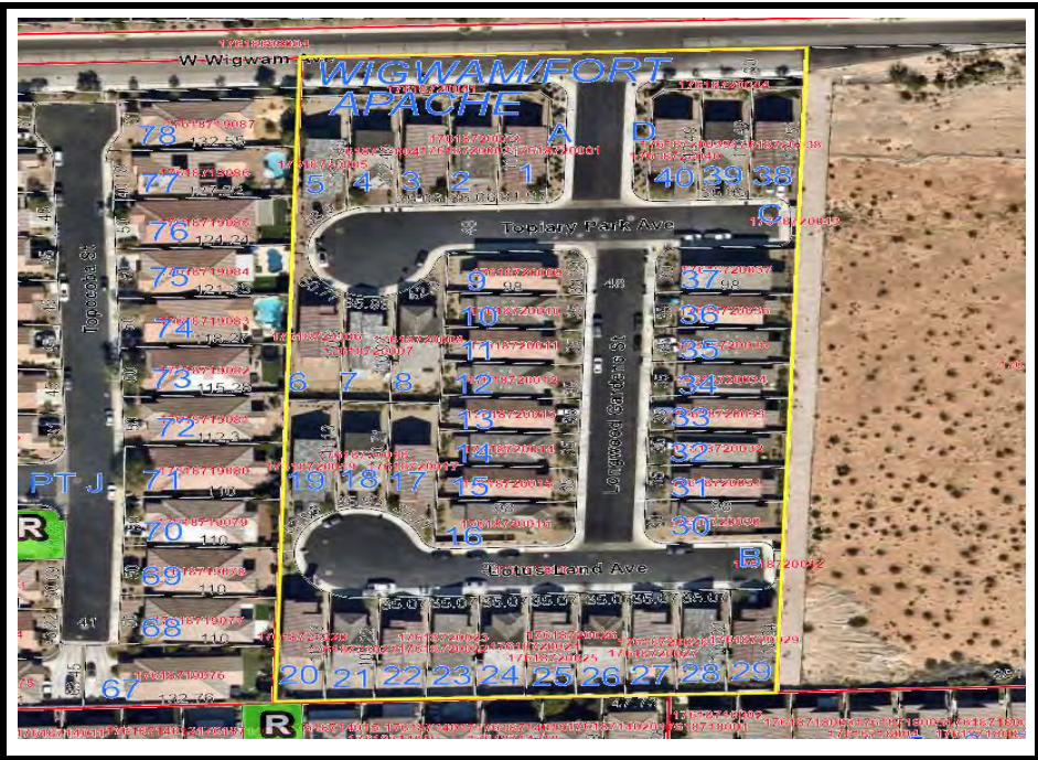
Subject Community Development Progress (10/2025) Aerial Photo
