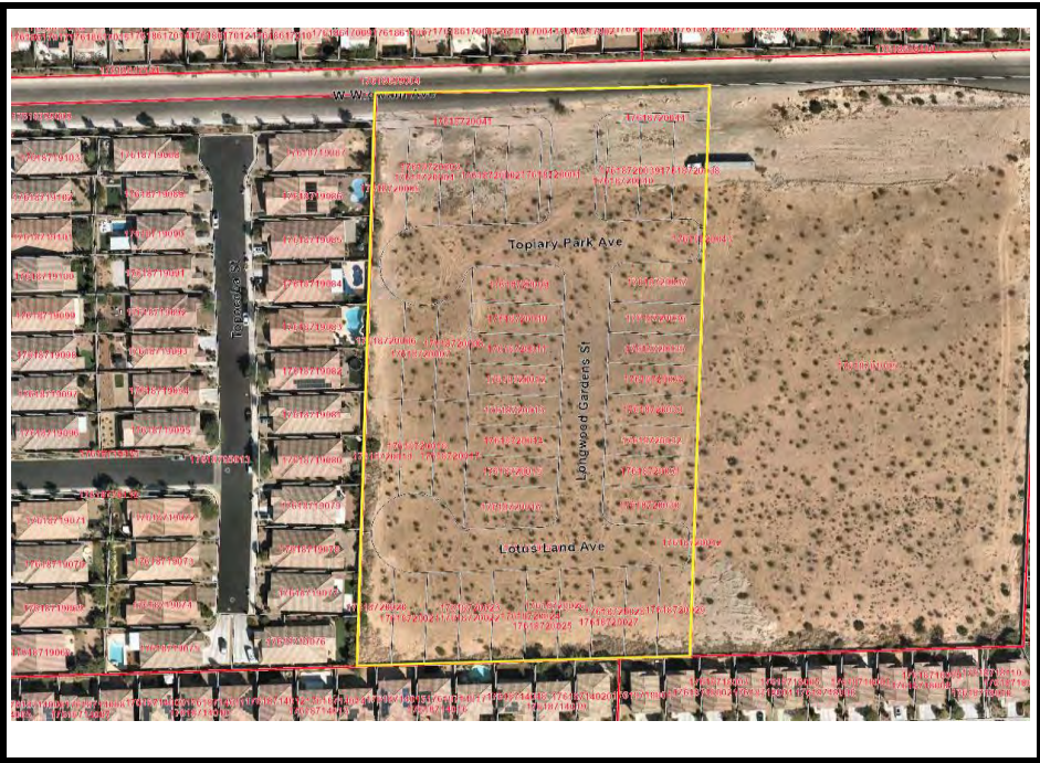
Subject Community (12/01/2021) Purchase Date (09/2021) Aerial Photo
